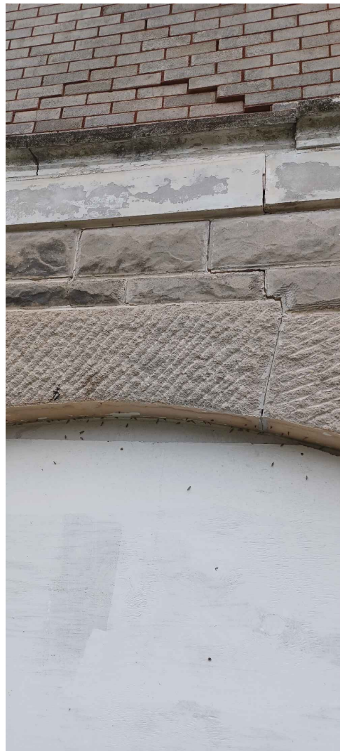
3 | DISPLACED BRICKS
